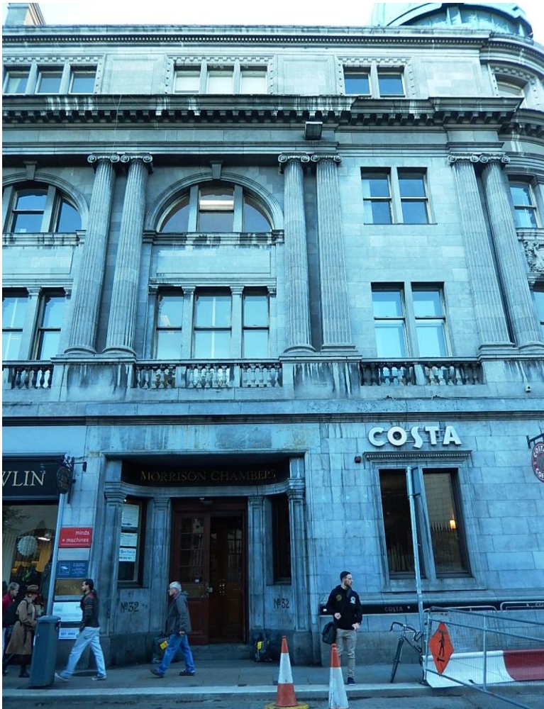
32-33 Nassau Street (Morrison Chambers)
